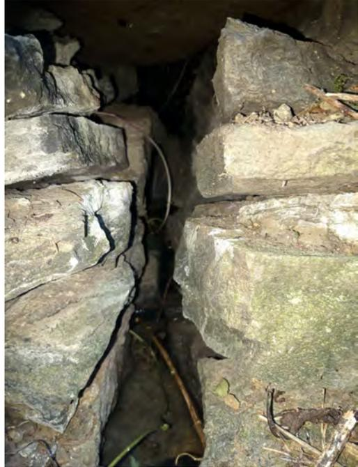
Photograph 15 - Inside the dry-stone outfall from Pipe B
